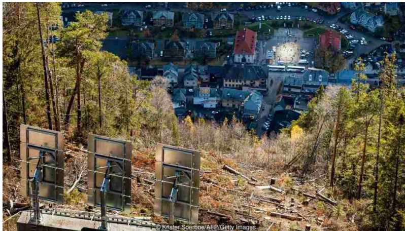
Figure 19 - Looking down on Rjukan, the path of the reflected sunlight [14].
