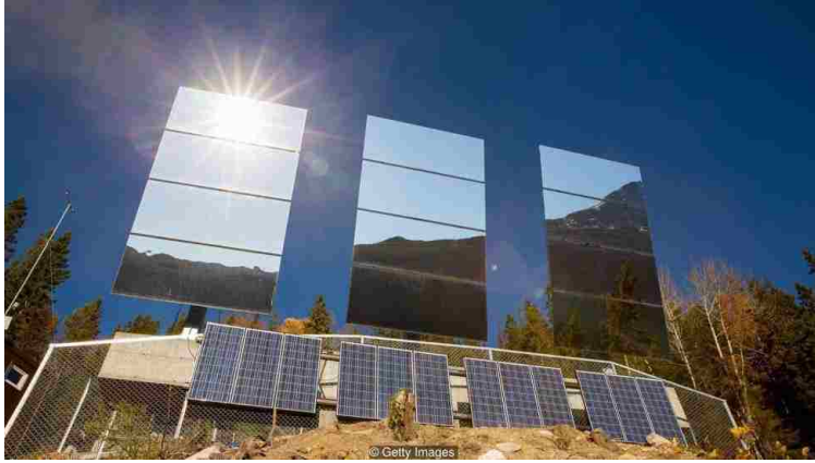
Figure 17 - The mirrors are mounted to keep track of the sun [14].
